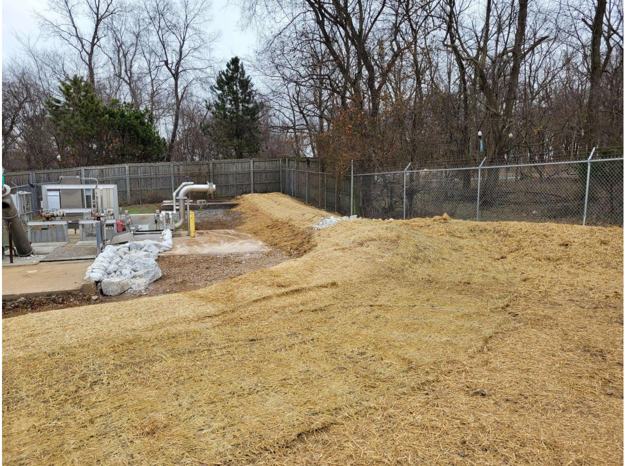
Completed berm construction on February 10 th , 2025 (2)
